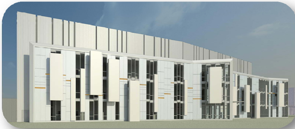
Figure 1 – Western Façade (All photos courtesy of Cannon Design)
